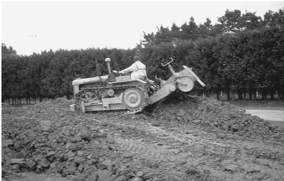
**Plate A1** Rotavation of clay fill
