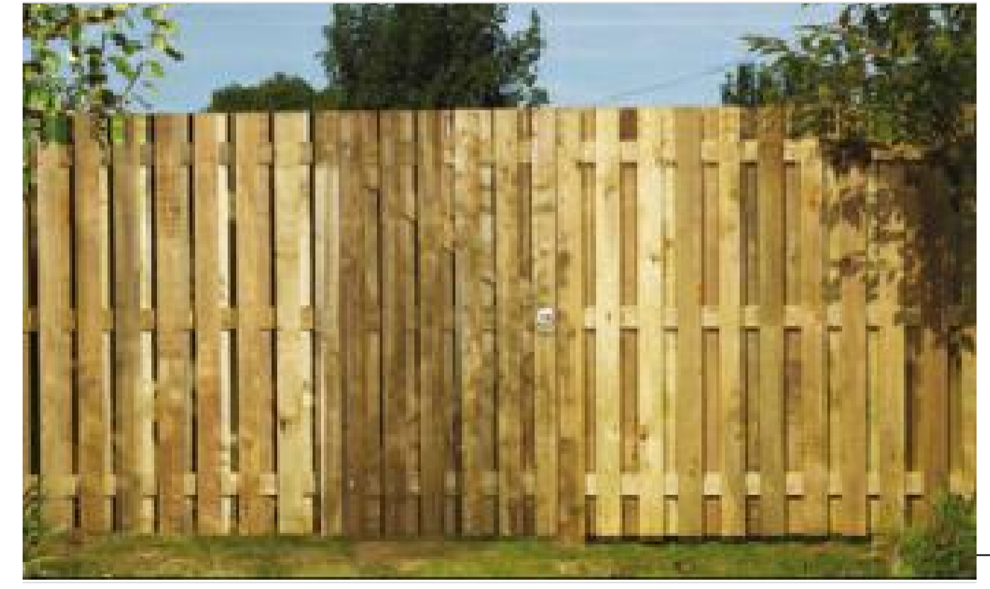
PHOTO OF TYPICAL HIT & MISS TIMBER FENCE
