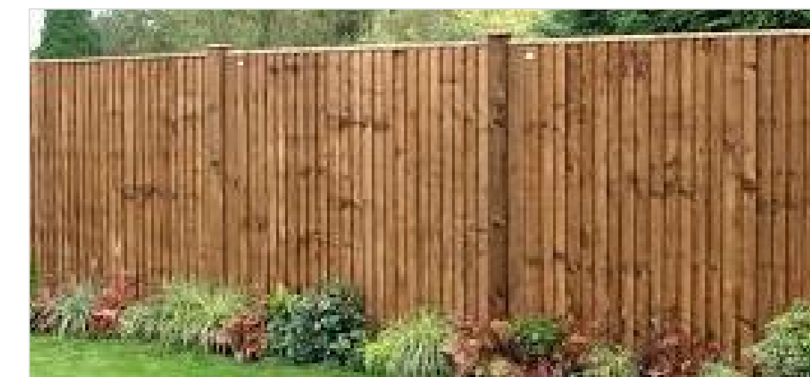
PHOTO OF TYPICAL CLOSEBOARDED TIMBER FENCE
