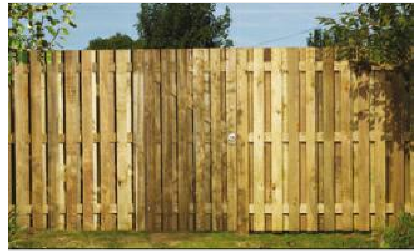
PHOTO OF TYPICAL HIT & MISS TIMBER FENCE
